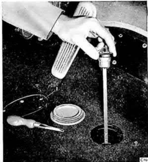
Fig 29 ACCESS TO THE GEARBOX DIPSTICK
